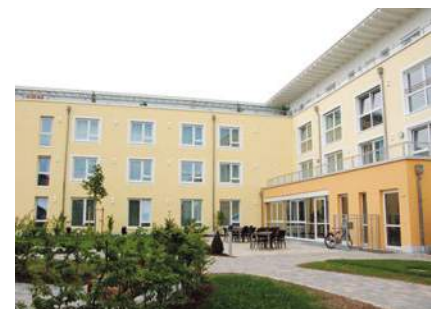
Regensburg-Burgweinting retirement home: centralised control of the M-WRG units and use of the cost-effective 2-room solution
